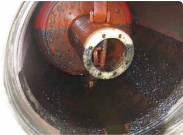
Figure 1. Result of pigging a “dry” network
